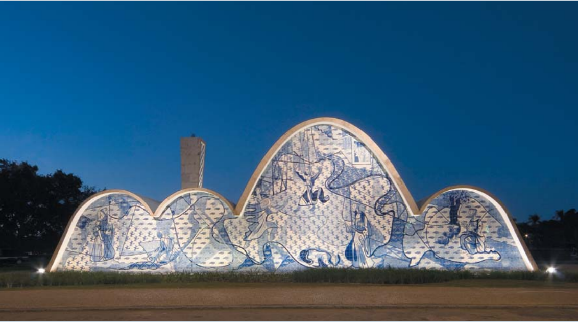
The rear facade of the church is decorated by a mosaic that depicts scenes from the life of St. Francis. Inground luminaires wash the wall with uniform light and render the work of art visible after dark – the eaves are outlined in light and form a frame for the picture.
