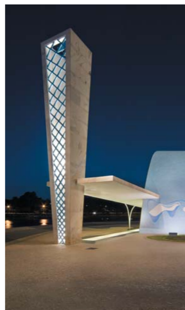
The bell tower stands as a separate element in front of the church. The church and the bell tower are linked via an awning and via light.
